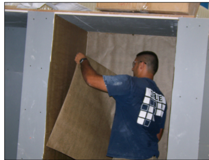
Applying waterproof barrier paper.
