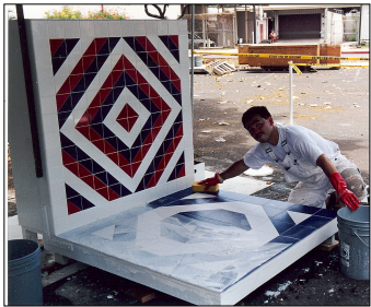
Finishing (grouting) tile work.
