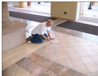
Replacing tiles, repairs.
